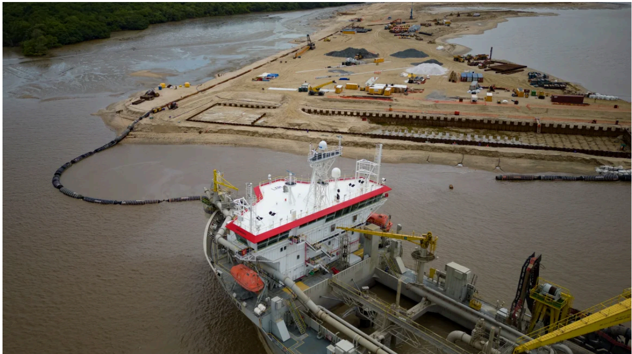
A ship creates an artificial island by extracting offshore sand to create a coastal port for offshore oil production at the mouth of the Demerara River in Georgetown, Guyana, Tuesday, April 11, 2023. [Matias Delacroix/AP]
